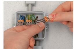
Strip solid conductor to 11 mm/0.43 inch (see marking).
